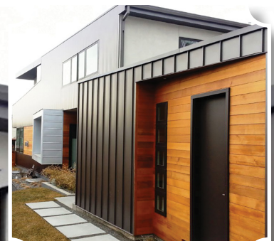
Vintage® Roof & Wall Project Completed by Z-Craft
